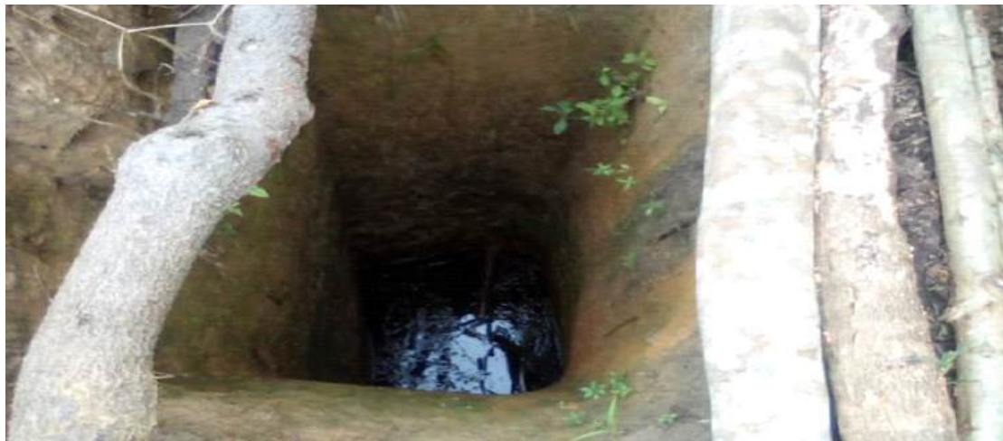
Plate 2: Shows the unsanitary condition of shallow hand dug system for RWH in the dry season.
