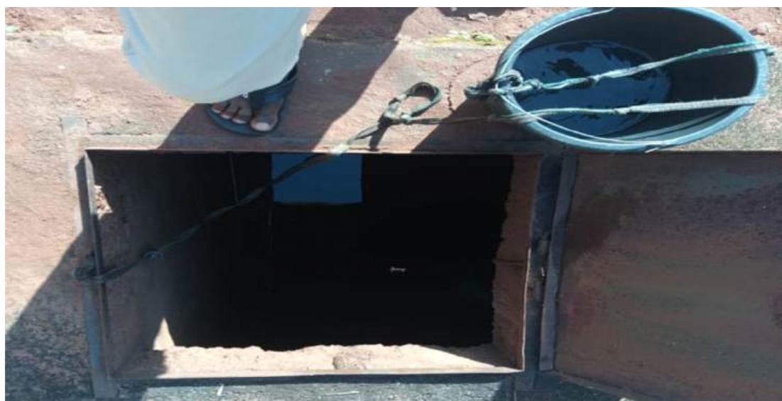
Plate 3: Shows a coverable underground well system built for RWH in the community.
