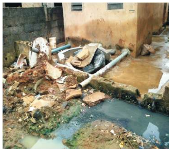
Figure 4: Toilet with sewage discharged into an open drain
