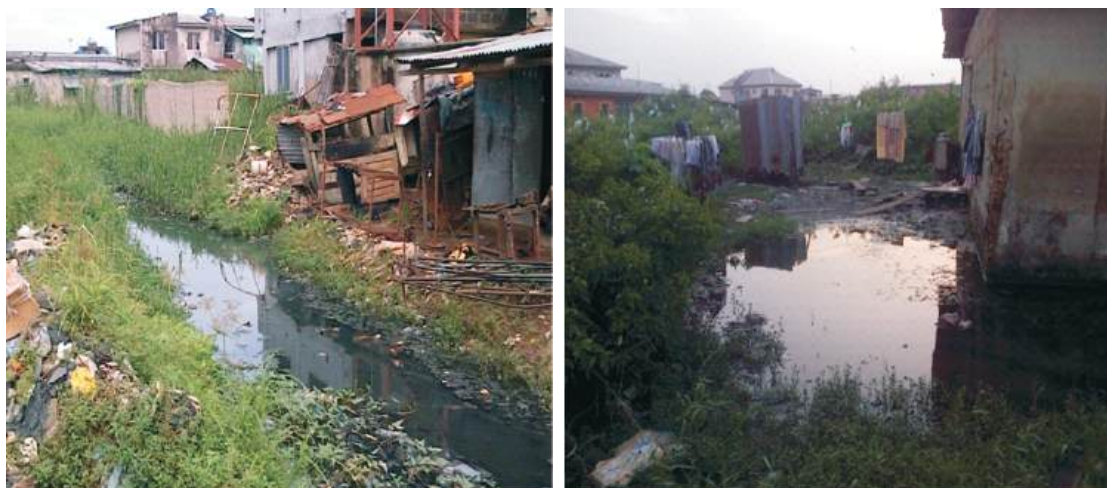
Figures 1a and b: Views of some residential buildings where the study took place
