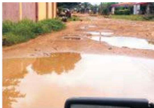
Plate 4: A flooded street with blocked gutters
