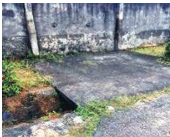
Plate 27: Water supply outlets from a residence
