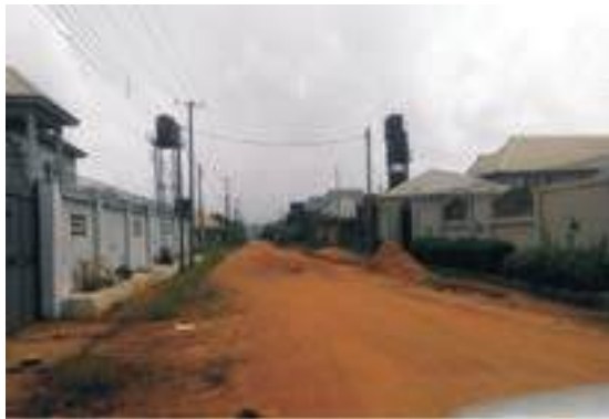
Plate 28: Earth road in the estate
